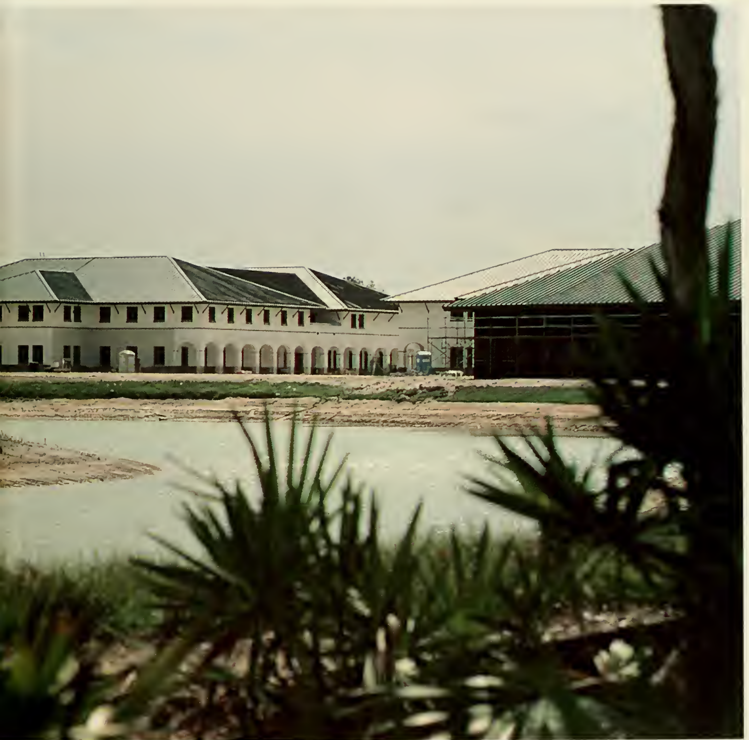
Dark green standing-seam metal roofing was chosen to create a "tree canopy" effect. Gray stucco exteriors are accented with brown, cast stone wainscots at ground level. Photograph: Gary Knight & Associates Photography.
